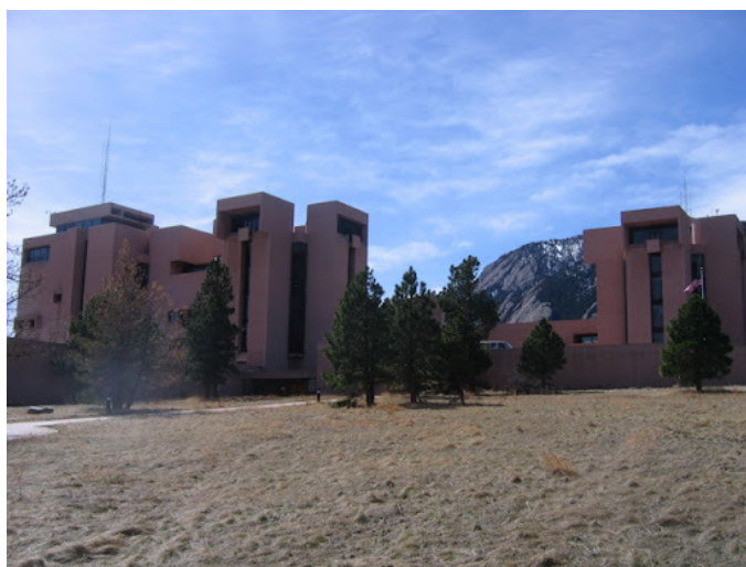
Figure 3: The National Center for Atmospheric Research (NCAR) in Boulder, Colorado.
